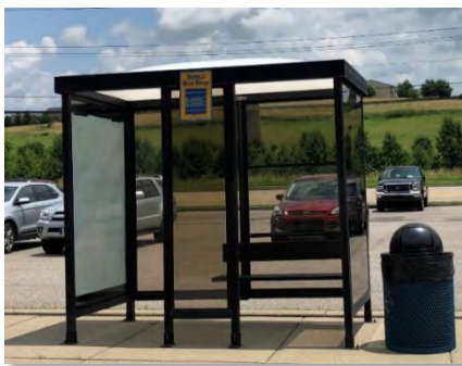
Figure 11-3: Empire Drive at Dixie Highway Shelter
